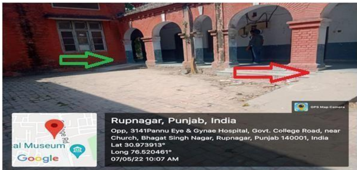
Ramps at the backside of Music Department
